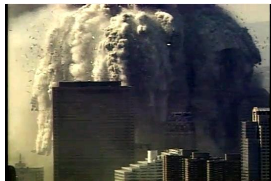
Note the large, free-flying steel framing sections, trailing smoke clouds, which landed hundreds of feet outside of the building's perimeter.
