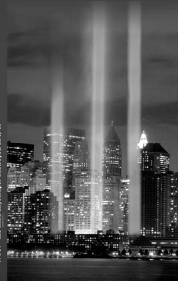
WTC7 - the third skyscraper destroyed on 9/11
